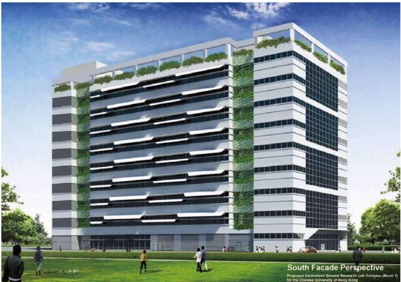
The exterior outlook of the new research building of the School of Biomedical Sciences
